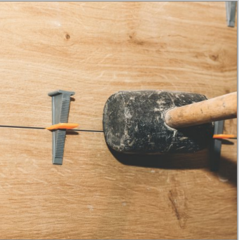
Remove Wedges Ones It Dry
