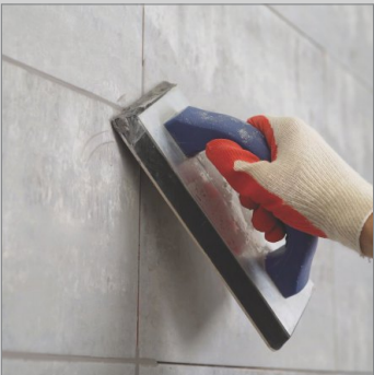
Joint Grouting
