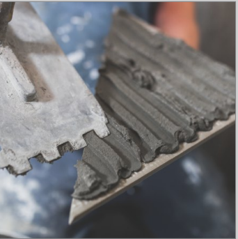
Cement Laying On Tile
