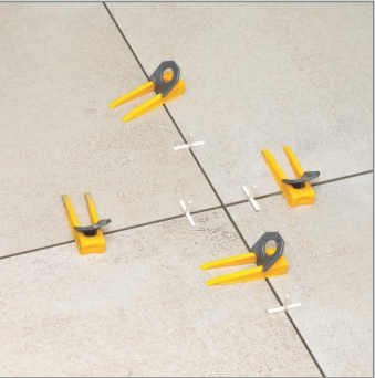
After Lavelling Process Leave Int For 8-10 Hrs.
