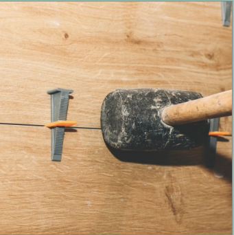
Remove Wedges Ones It Dry
