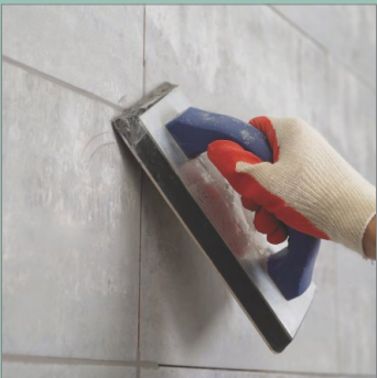
Joint Grouting
