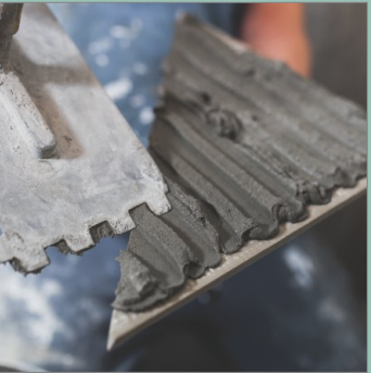
Cement Laying On Tile
