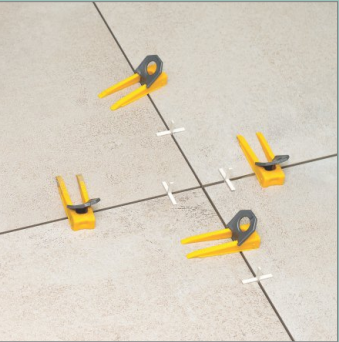
After Lavelling Process Leave Int For 8-10 Hrs.
